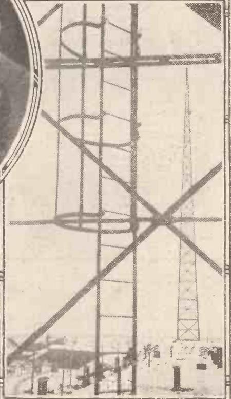
A close-up of the ladder and guard which run from the ground to the tops of the masts.
