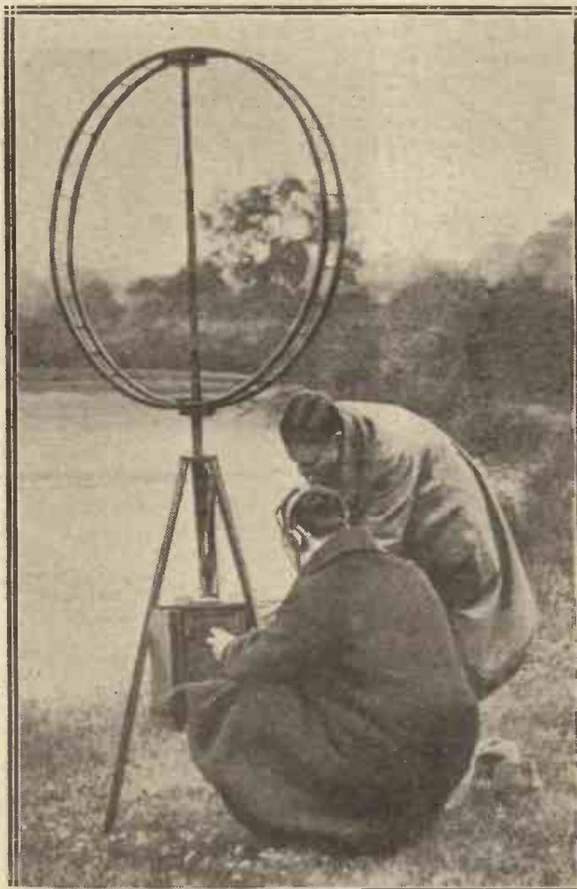
Direction Finding with Portable Receivers. Members of the Golder's Green and Hendon Radio Society are shown taking wireless bearings from a hidden transmitter.
