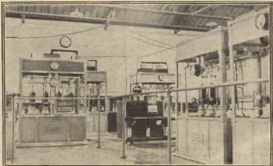
A general view of some of the transmitter units at 5 X X. To the right are the modulating panels, the oscillating panels being in the background.
