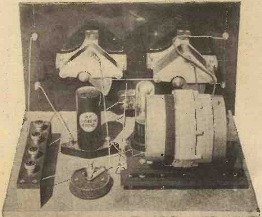
A general view of the interior of the All-Wave Reinartz One-Valver, ready for placing into its cabinet.
