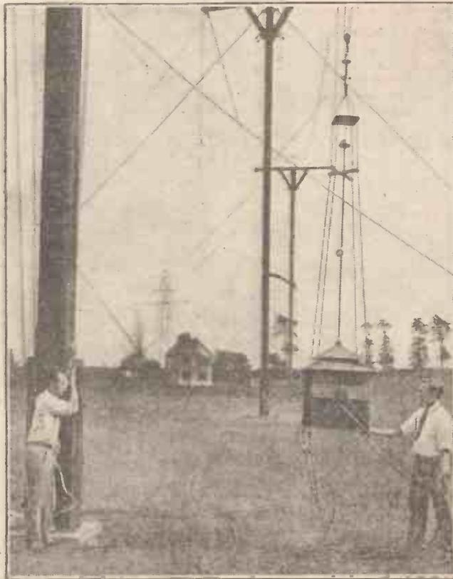
American engineers hoisting a 5 metre transmitter up its mast, where it operates 75 feet from the ground. The meter on the instrument is read with the aid of a telescope.
