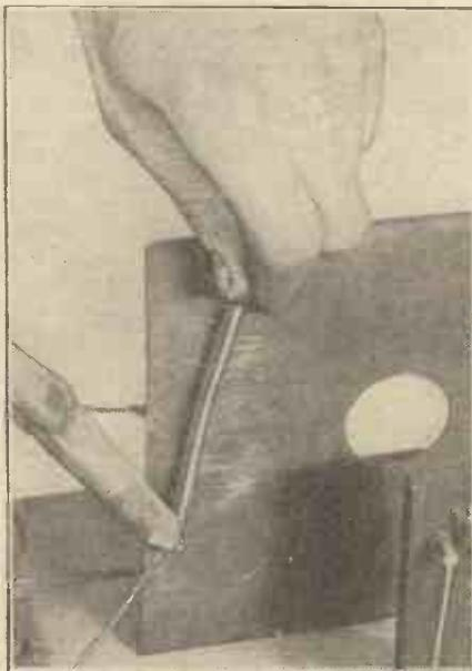
The solder should be placed in contact with the iron and the metals to be soldered, when a big joint is to be made.
