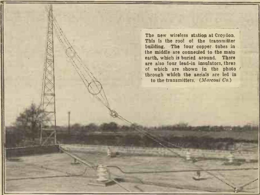
The new wireless station at Croydon. This is the roof of the transmitter building. The four copper tubes in the middle are connected to the main earth, which is buried around. There are also four lead-in insulators, three of which are shown in the photo through which the aerials are led in to the transmitters. (Marconi Co.)
