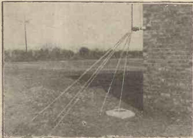
One of the features of the new wireless station which serves the Croydon Aerodrome is a very complete and efficient earthing system. The connecting wires shown in the above photo are joined to a large buried earth ring which surrounds the station.
