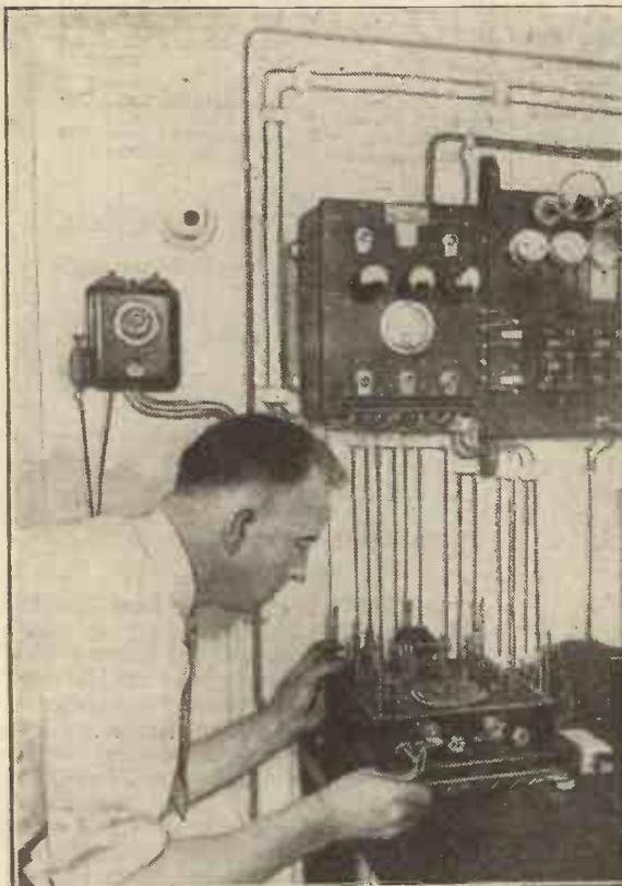
This operator is adjusting a ship's "automatic listener," which keeps a wireless watch for distress calls even when no operator is listening-in. All ordinary calls are ignored by the selector device, but if an SOS comes along it rings bells in the operator's cabin, in the radio-room, and on the bridge.
