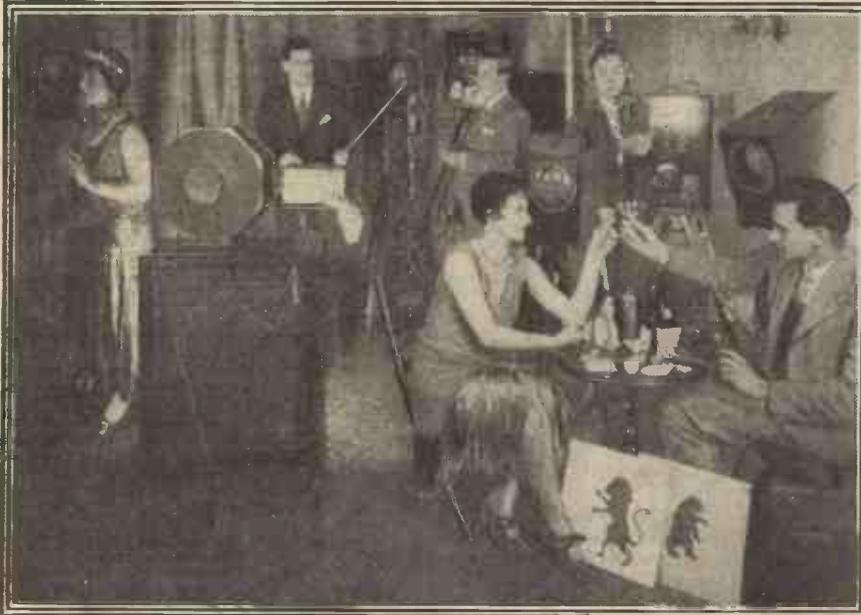
A most elaborate scheme was recently framed in connection with an American Television experiment. In order merely to "get over" simple objects, such as hands and revolvers in outline, to illustrate a radio drama, three television transmitters were used.
