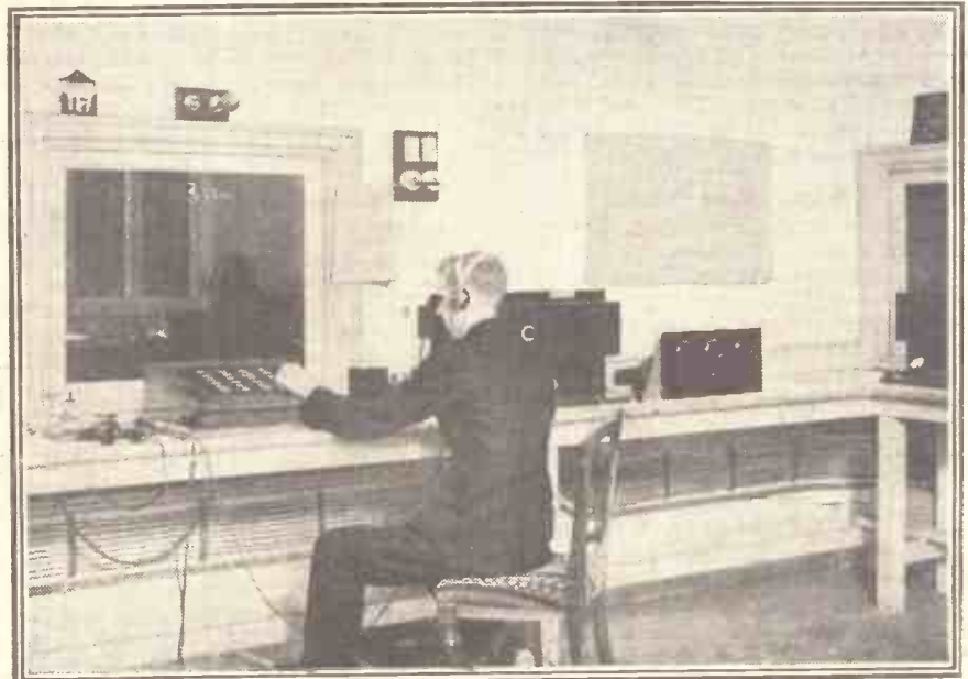
Checking the broadcast transmission from the control room at Dublin, 2 R N.
