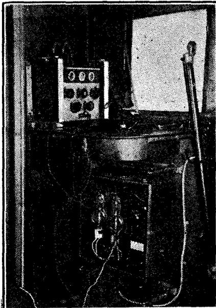
The radio gear installed on the “Yellow Bird,” the aeroplane in which three brave Frenchmen flew the Atlantic from West to East.
