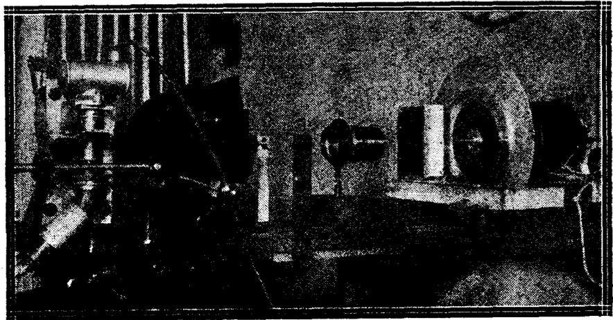
The film is run through the small projector on the left, and the image is focussed through the lens to the sensitive cell on the other side of the scanning disc.
