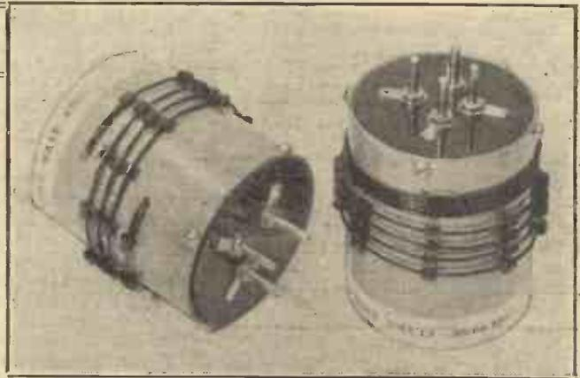
Two interesting short-wave coils produced by Messrs. Ward & Goldstone. Note the method of spacing the aerial winding.
