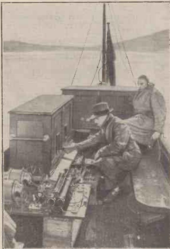
The B.B.C. launch, "Magician," which is fitted with a complete transmitting outfit for passing on boat-race and other river commentaries.
