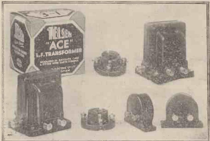
This photo shows two each of the new Telsen transformer, H.F. choke and valve holder.
