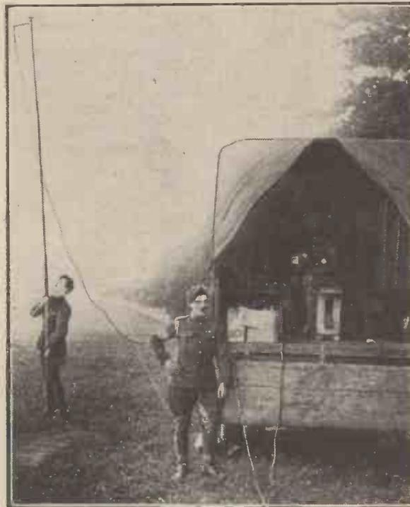
Having plenty of spare vans and petrol, the Army's idea of a "portable" set is one which can go into a big lorry, that also carries collapsible masts and a signalling crew. This view shows a field wireless set just going into action near Cheltenham.
