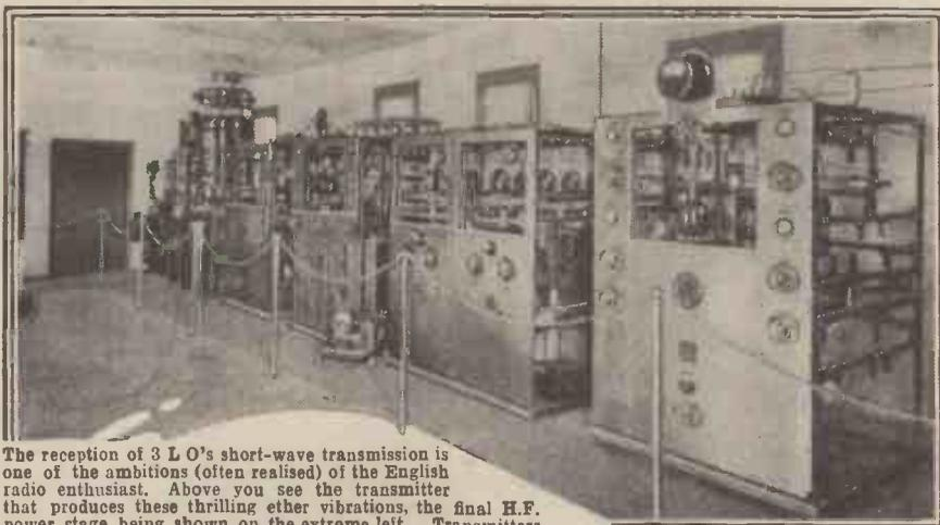
The reception of 3 L O's short-wave transmission is one of the ambitions (often realised) of the English radio enthusiast. Above you see the transmitter that produces these thrilling ether vibrations, the final H.F. power stage being shown on the extreme left. Transmitters use H.F. amplifiers very similar to receivers. The energy in this case is modulated with speech and music, and then amplified at H.F. until sufficient aerial power is developed.
