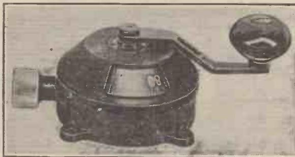
A new radio-set tuning device for aeroplanes. The pilot merely has to knock the handle round with his gloved hand to tune his radio outfit.
