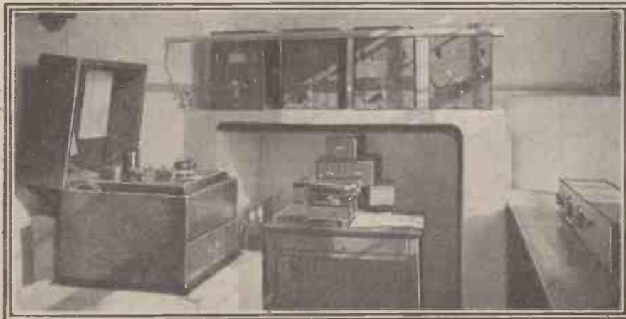
Here you see the very specially calibrated wave-meters at Tatsfield, where B.B.C. engineers check the transmissions, and where they pick up the programmes of distant stations for relaying to British listeners.
