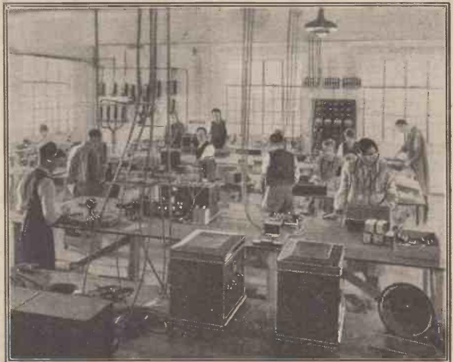
The testing laboratory of Messrs. Radio Instruments Ltd., where completed receivers are put through their paces before being placed in their cabinets and sent off for distribution to the public.
