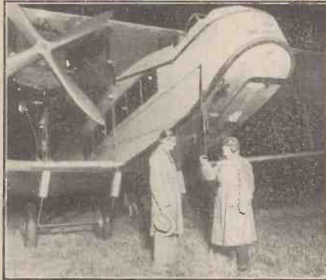
This picture shows Capt. Brewer, the B.B.C. commentator, talking to Capt. Spafford, the pilot of the "City of Melbourne," before the recent night broadcast from the air. The pilot is holding the plane's aerial, from which the commentary was radiated, and as soon as the broadcast was over the plane proceeded to Croydon without descending.
