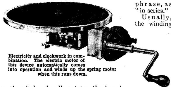
Electricity and clockwork in combination. The electric motor of this device automatically comes into operation and winds up the spring motor when this runs down.
