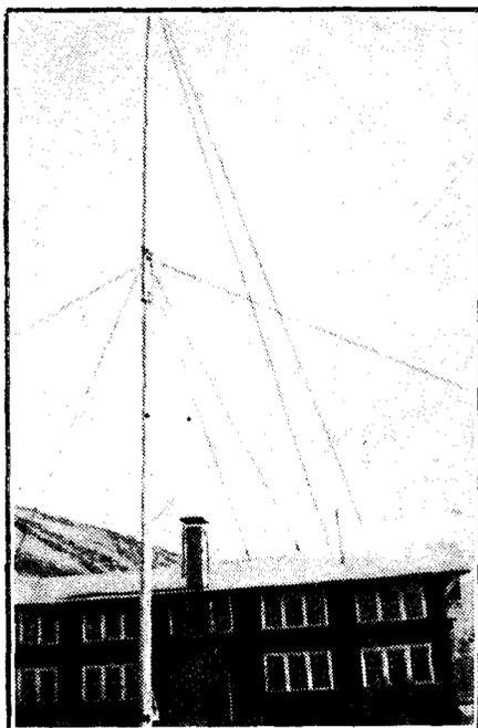
The aerial at K U O M is of the simplest kind, and is fixed between two wooden masts, but its radiation efficiency is excellent.
