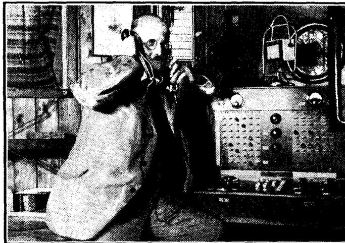
Dr. W. Reisser, at the Zehlendorff laboratory, testing a system by means of which he can interpose announcements in a relayed programme, and at the same time hear the programme before and after relaying.
