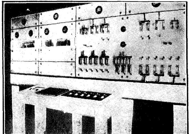
The studio at K U O M and the main switchboard. Between these two the energy representing the speech and music is amplified millions of times by valve magnifiers.
