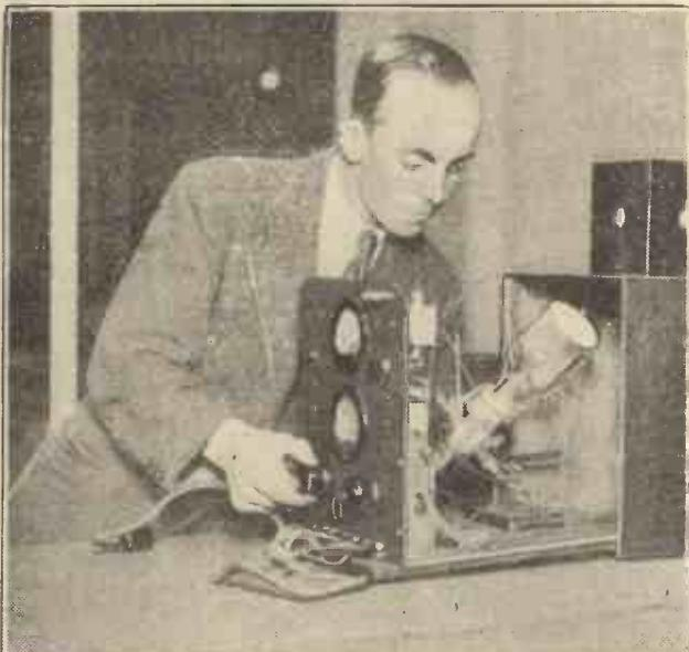
This newly-invented "Navigation Compass" is for use by ships in fog, and is sensitive to sound waves and warning signals.
