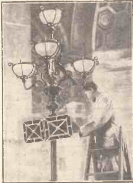
Putting the final touches to some of the loud speakers that have been installed in St. Paul's Cathedral to enable everyone to hear the service.
