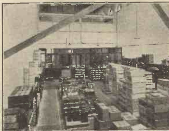
A corner of the new "Exide" accumulator store opened at Bristol by the Chloride Electrical Co. Ltd.
