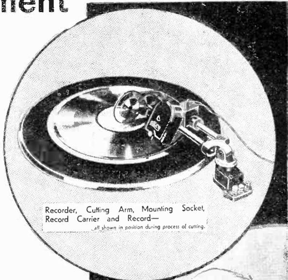
Recorder, Cutting Arm, Mounting Socket, Record Carrier and Record—
