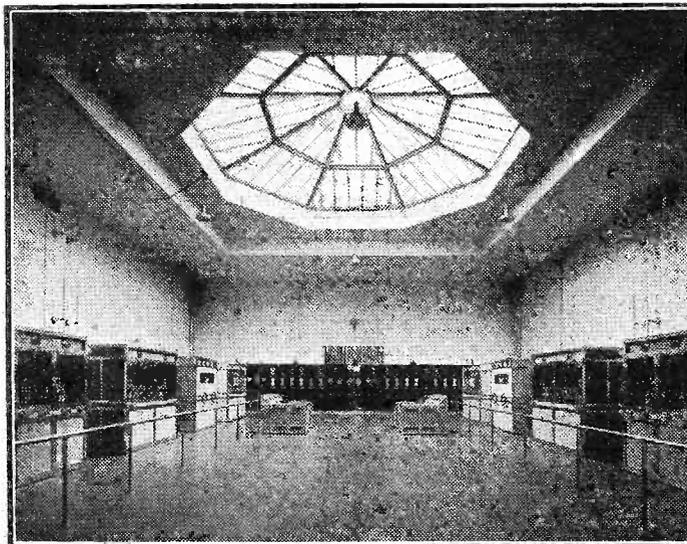
This excellent view of the transmitter hall shows the floodlighting dome, 30 ft. above the ground, which provides all the illumination for the control engineers without any glare. The floor is made of compressed cork, a new material for this purpose.
