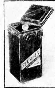
The new "Block" battery is of unique construction. It has one substantial block of active material, the interior of the casing acting as the other electrode.
