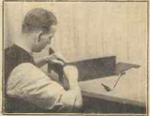
Fig. 2. The first stage in assembling the "Easy-Cabinet." Fixing the left-hand side-piece to the top.
