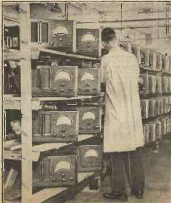
This is a corner of what is known as the "soak" testing department at the H.M.V. works. Up to 1,000 receivers can be played simultaneously.
