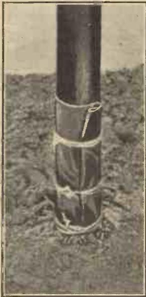
Rubber tubing bound round the earth tube, and well covering the point of entry to the ground, will prevent corrosion.
