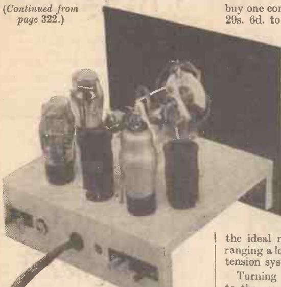
A four-valve short-wave set made up from one of the Peto-Scott "Pilot" Experimenter Kits, using a standard chassis and baseboard.
