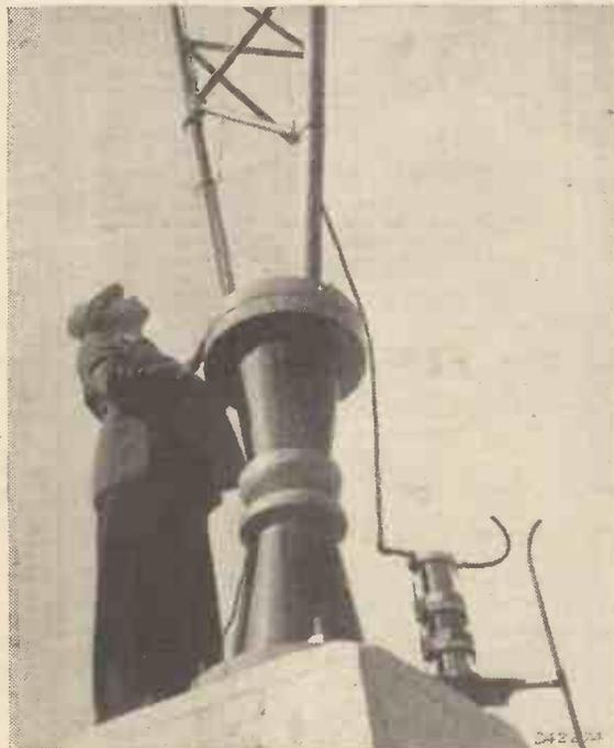
Though weighing 60 tons, the new aerial mast at KDKA, the well-known American station, rests on a porcelain insulator base about 3 feet high and 18 inches in diameter. Mr. H. W. Irving, of the Westinghouse Company, is seen here looking up the mast, which is 718 feet high.
