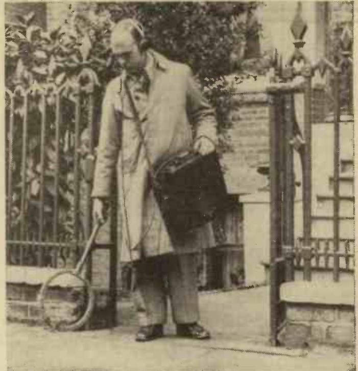
All complaints of interference are investigated by a special G.P.O. squad who are equipped with suitable trouble-tracking apparatus. Here is one of the G.P.O. experts with a portable set and small interference-locating aerial.
