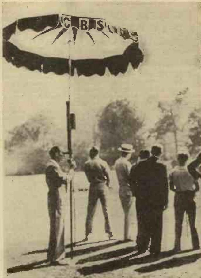
An ingenious scheme instituted by the Columbia Broadcasting System of America to facilitate outside broadcasts. The weird-looking arrangement with the sunshade on top is a telescopic periscope with which the commentator is able to see over the heads of spectators. The "mike" is fitted just below the periscope eye-piece.
