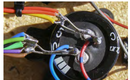
Fig.27. Nodding on a power supply capacitor. The lower left cable cluster contains the ground cables/stub; the upper left contains the power cables/stub.
