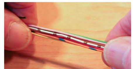
Fig.3. Relieving the tension and straightening out the loom.
