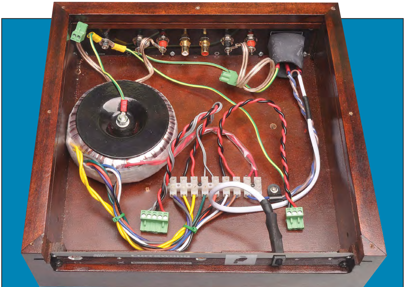
The new transformer mounted inside the same plinth which held the original two transformers. Again, ensure that any exposed mains wiring (for example, the IEC mains input socket) is properly covered, as shown here.
