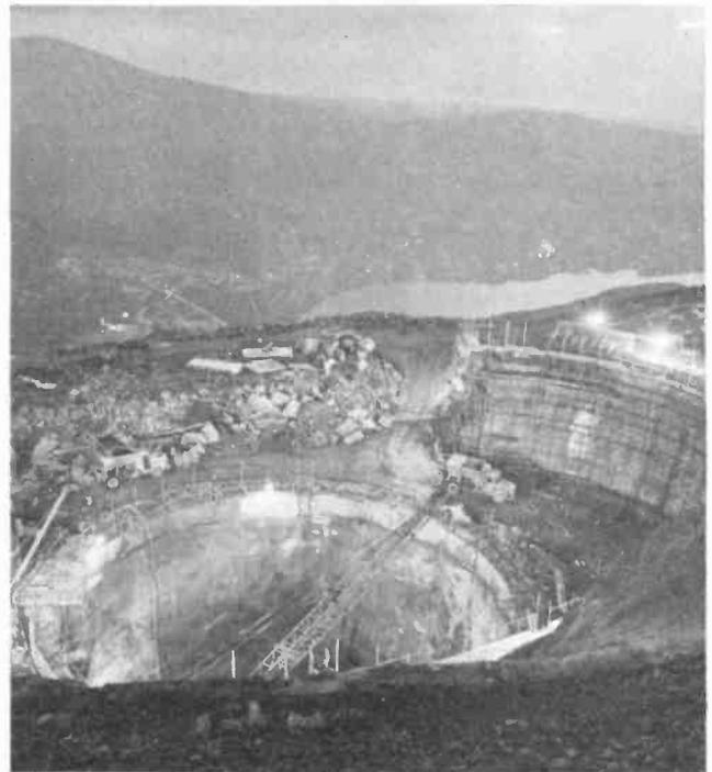
The surge-shaft under construction. 584 metres below this point the water from Marchlyn reservoir enters the high-pressure feed tunnel
