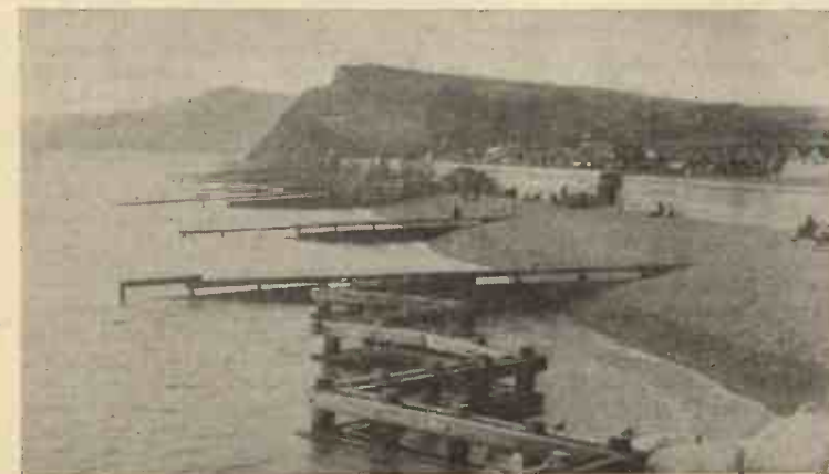
Breakwaters and groynes, West Bay, Bridport.
