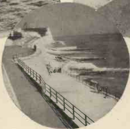
A simple type of seawall at Teignmouth.
