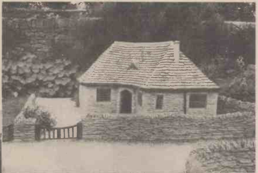
A Cotswold bungalow with walls built "in courses" and a garden wall built in the Cotswold manner, without cement
