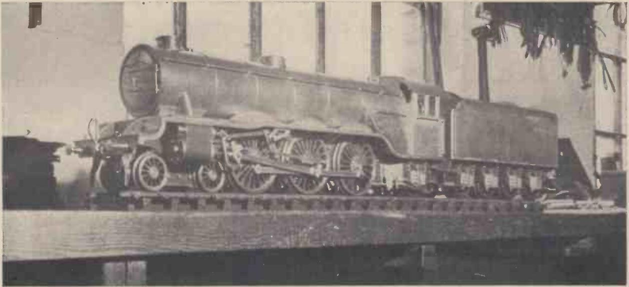
Fig. 1.—A picture of our 2½ in. scale model of the famous L.N.E.R. "Flying Scotsman"
