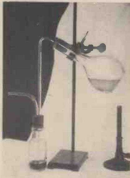
Preparing bromine by heating a mixture of potash bromide, manganese dioxide and concentrated sulphur. The bromine distils over as a heavy red vapour condenses in the bottle
