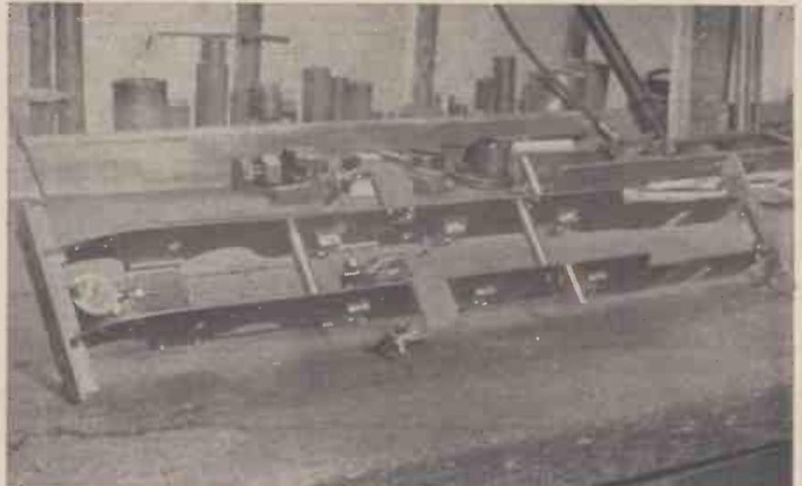
Fig. 10.—The finished main frames with buffer beams and displacement lubricator in position
