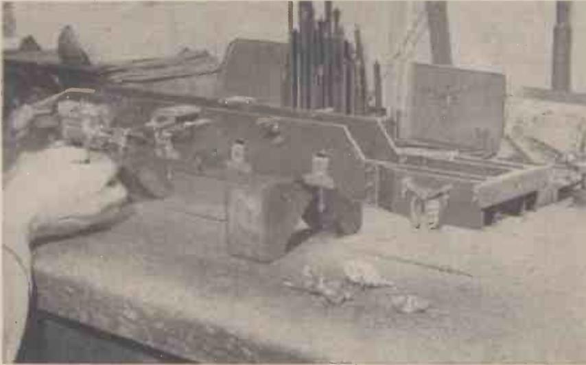
Fig. 9.—The main frames, showing one of the cylinders being fitted
