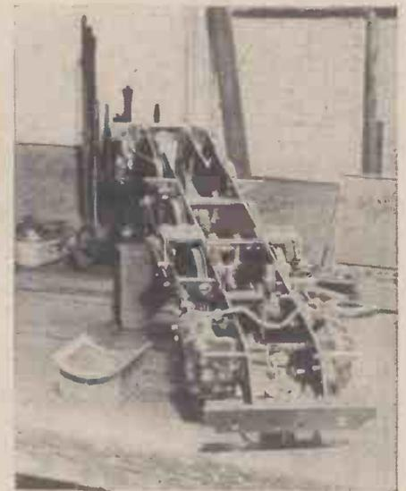
Fig. 23.—This view of the engine chassis shows the steam and exhaust pipe connections, feed pump, and footplate brackets
