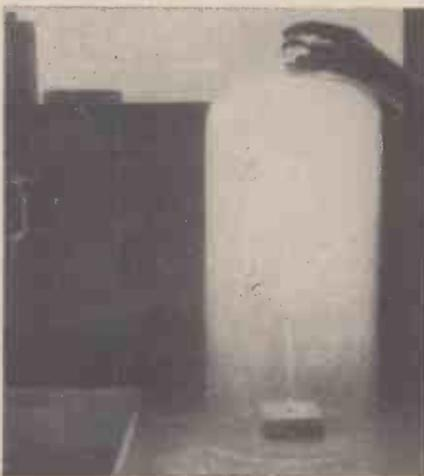
Preparing phosphorus pentoxide by burning phosphorus in air under a large bell jar. The white clouds of the pentoxide collect as a deposit on the inner side of the jar
