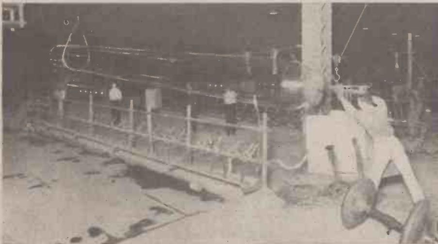
Fig. 3. Lowering on to the rest for cutting up into lengths. The glass cylinder illustrated measures 35 ft. in length by 36 ins. diameter.
