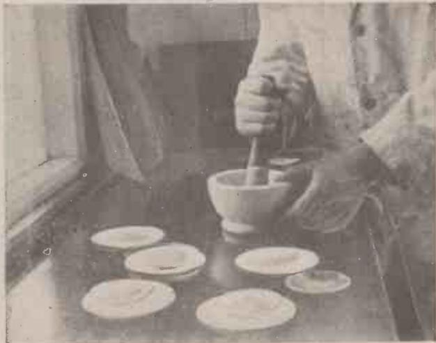
Grinding pigments into "colour bases" for the shading of cosmetic powders.
