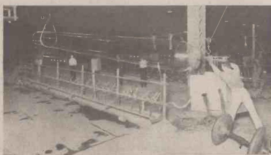
Fig. 3. Lowering on to the rest for cutting up into lengths. The glass cylinder illustrated measures 35 ft. in length by 36 ins. diameter.
