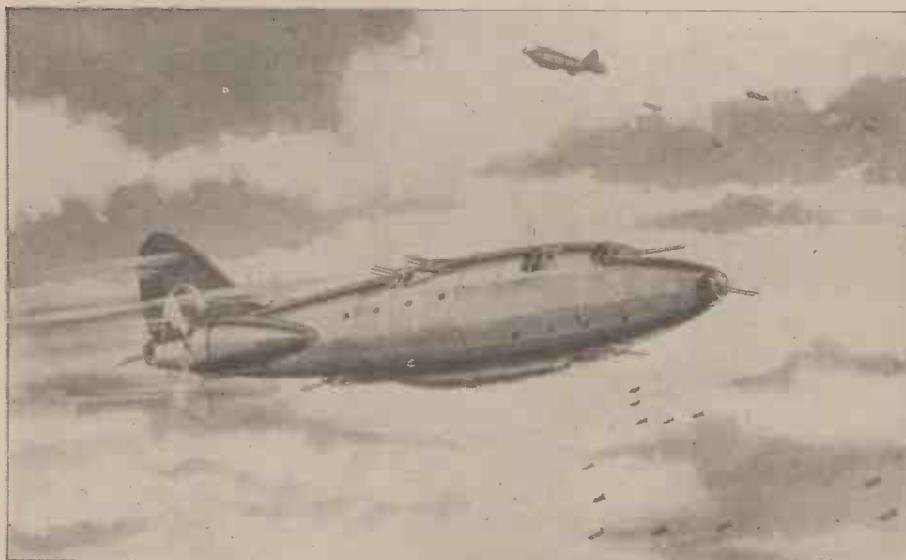
As the inventor sees the heavily armoured and gunned 100-ton aerial tank of the future, with 2,000 h.p. enclosed lift engines, dynamos, and radiators, and two 1,000 h.p. pusher propelling engines.
