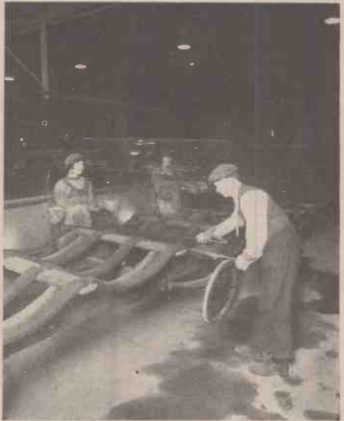
Fig. 4. A section of a glass cylinder being split into "shawls" before flattening.
