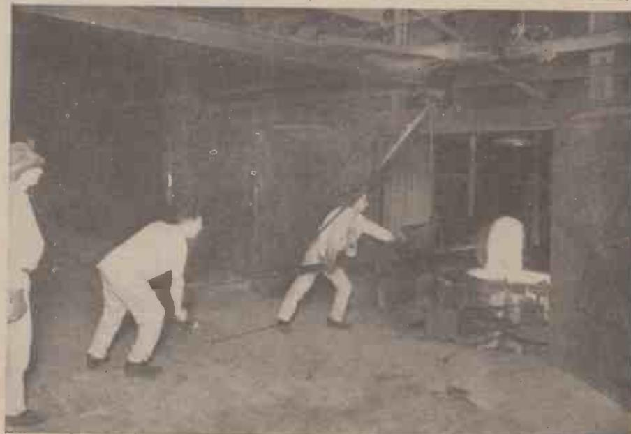
Fig. 1. Teeming the molten glass into the double-sided crucible, or drawing pot.
