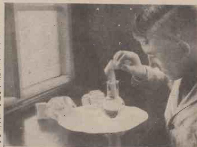
*The first stage in the making of nail varnish. Preparing the celluloid solution by dissolving scrap celluloid in an appropriate solvent*
