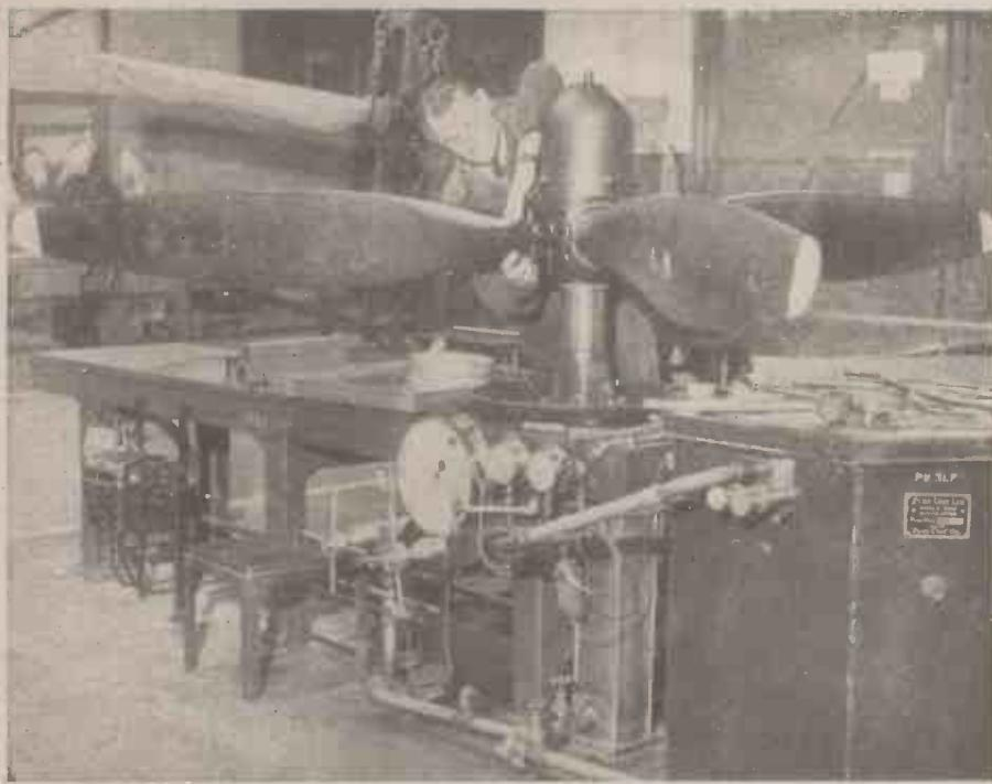
*Aeroplane propellers receiving the final test before despatch. The propeller is being tested in a factory which constructs these essential aircraft parts.*
