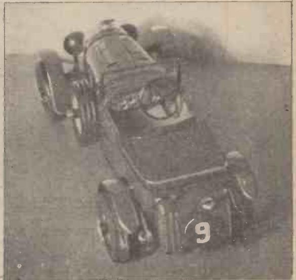
View of an unfinished model 4 1/2 litre Bentley, showing instrument panel, tank, etc. Note headlamps made from bulbs of "Ephedrine" droppers.
