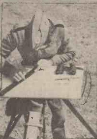
(Above) The plane-tableter plots a point of detail with the aid of his sight-rule. This is a most important task, for upon its accuracy the success of operations depended.
