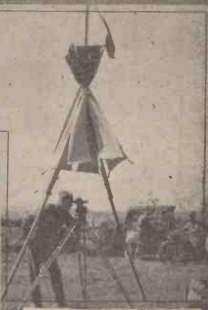
The field surveyor observing angles. The "booker" is alongside, writing down the readings, which when ready will be taken to the computing centre by the motor cyclist who has just arrived. The beacon, centred above the theodolite, is the target on to which the surveyors at other points observe.
