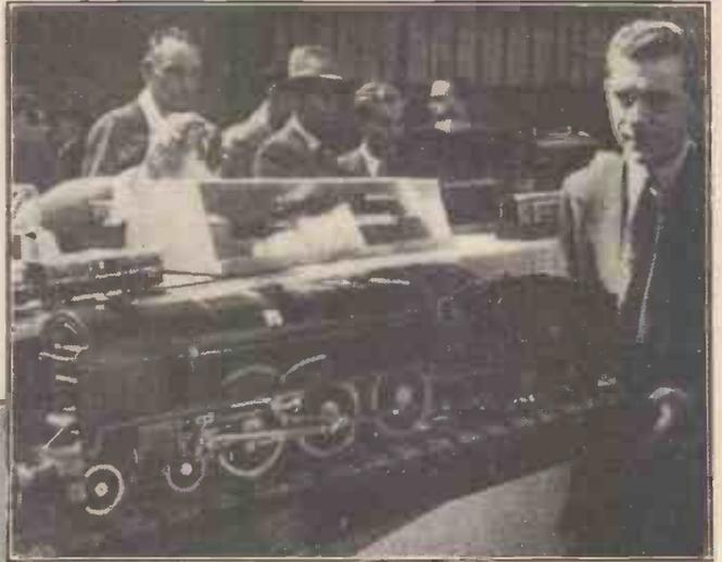
Fig. 4.—A much-admired L.M.S. model locomotive, made by Mr. G. Archer, apprentices' instructor at Percival Aircraft, Ltd., of Luton. The locomotive is a  $3\frac{1}{2}$  in. gauge,  $\frac{1}{16}$  in. scale model of the L.M.S. "Royal Scot." The detail in this model was very carefully carried out, and was much appreciated by model railway builders.
