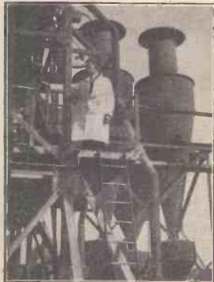
An oil-extraction plant of a type which may ultimately be used in the large-scale purification of synthetic fats or fatty acid products.
