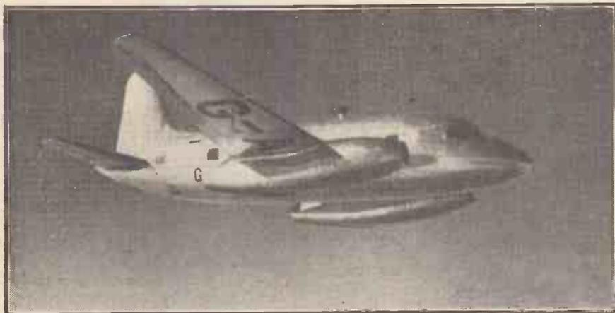
Fig. 4.—The Nene-powered experimental Viking.
