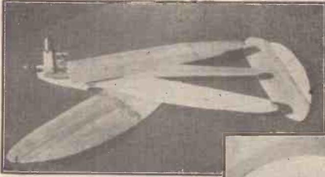
Fig. 29.—Solid block balsa is used for this little model's fuselage. Top and bottom are cemented on to a central crutch.
