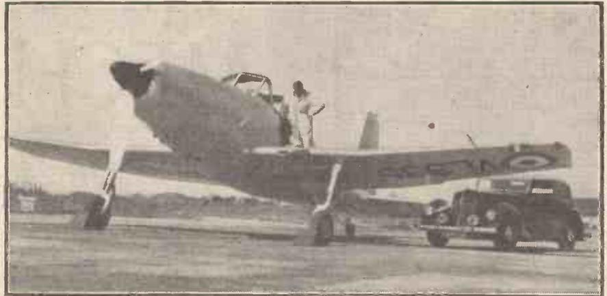
Armstrong Siddeley's Chief Test Pilot Sq. Ldr. Price-Owen, immediately before flying the Mamba gas turbine engined Balliol Trainer. The car bonnet housing a 16 h.p. engine is an interesting contrast in size with the nose of the aircraft housing the 1,000 h.p. Mamba, which incidentally weighs only 1,000lb. against the car's 3,000lb.
