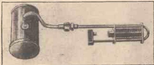
The Paraflame Burner and fuel container, made by Bassett-Lowke, Ltd.
