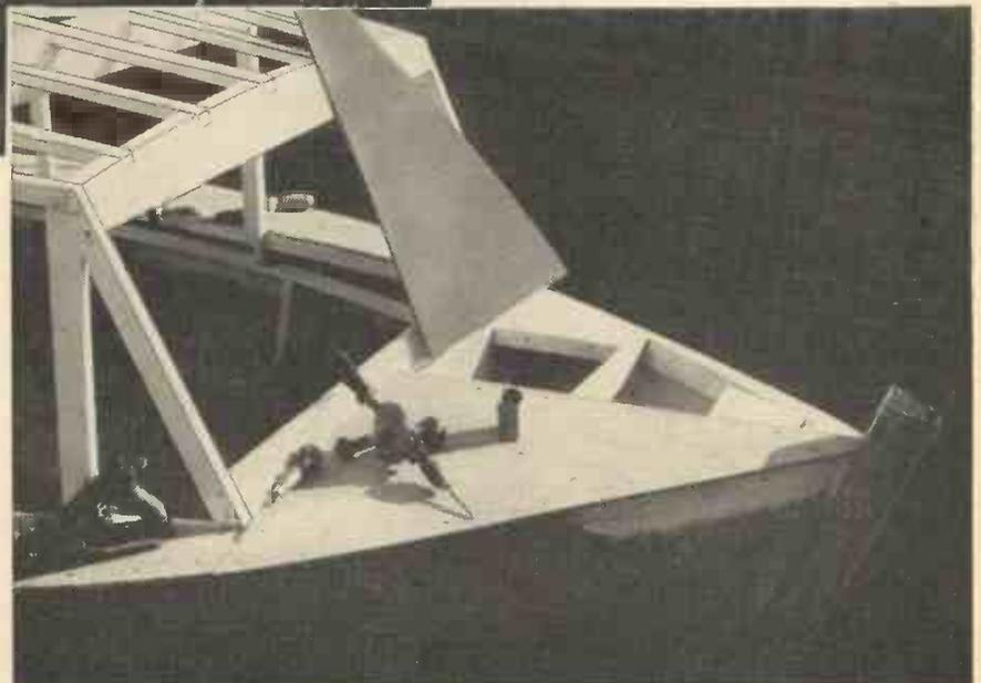
Fig. 31.—Fitting the fore-deck.
