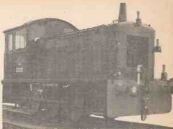
204 h.p. diesel mechanical shunting locomotive. Photo: British Railways.
