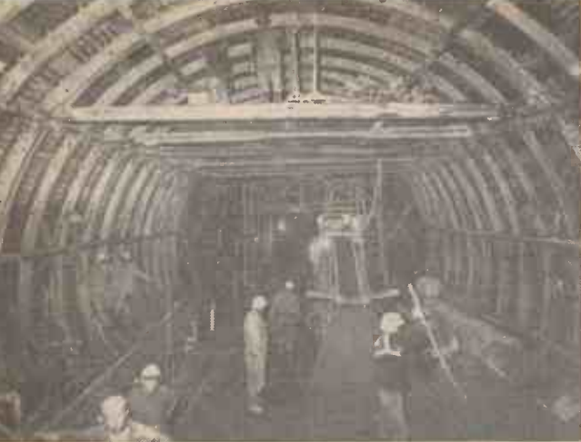
Fig. 6.—Work in progress deep inside the St. Bernard Massif.
