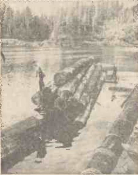
(top right) As the skidder brings a load of logs down to the water, the track-loader is transferring the previous load to the cradle. Note how the track-loader is guyed from the top of the A-frame to the raft. The centre-mounted A-frame permits guying without interfering with the swinging of the loader. The partially filled cradle is located in the left foreground beneath the water.
