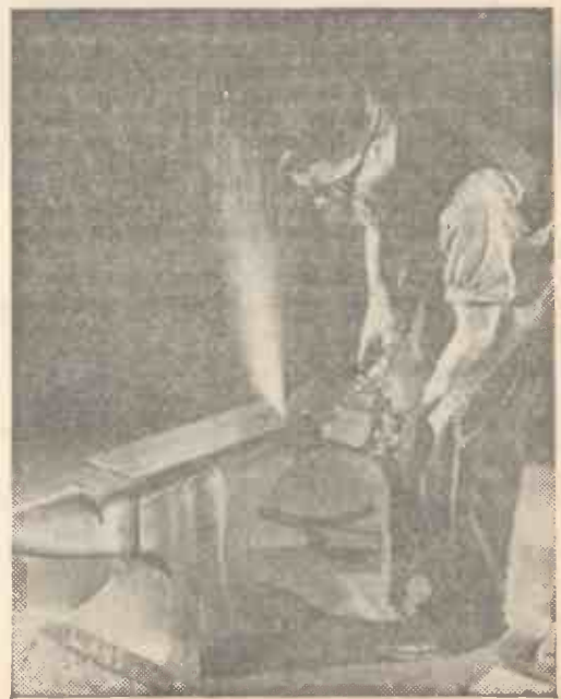
Fig. 8—Finish grinding an anvil.
