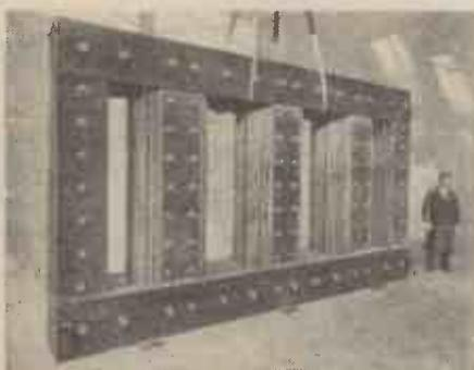
Fig. III. The core of the transformer
