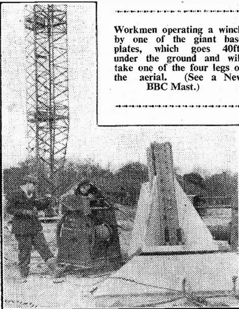
Workmen operating a winch by one of the giant base plates, which goes 40ft. under the ground and will take one of the four legs of the aerial. (See a New BBC Mast.)
