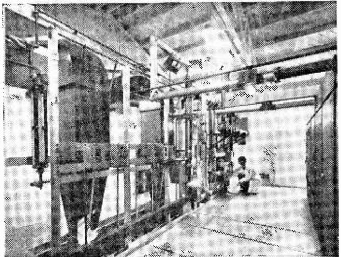
The combining unit and vestigial sideband filter assembly in the transmitter hall of the New Zealand Broadcasting Service's Channel 3 station at Christchurch which has been equipped by Marconi's Wireless Telegraph Co. Ltd.
