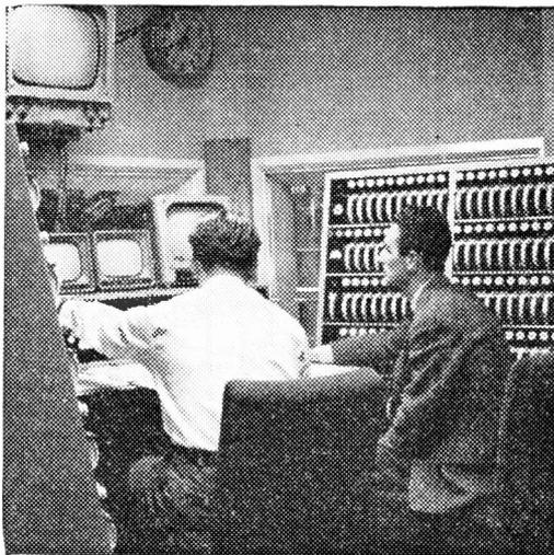
*A lighting supervisor at his console: he can view the output of each camera on the monitors in front of him to balance the lighting for each scene. ATV photo.*
