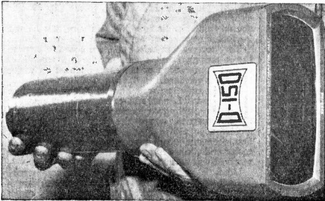
Lens for the D-150 incorporating backing lens of 5 1/2 in. f11.9.
