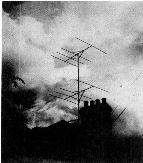
*In the final installation the double-four stacked array shown here was used for the ch. F2 vision. This was erected on an 18ft. mast and used cut down versions of ch. B2 arrays. The separate sound aerial is mounted on another chimney.*
