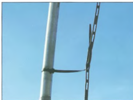
Fig. 4: Nylon ties hold the ladder line about 125mm from mast.
