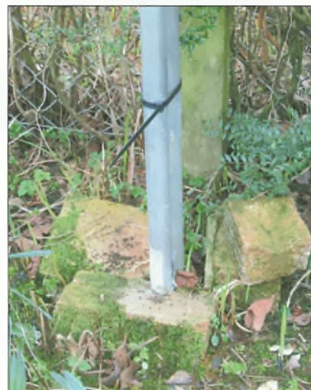
Base of mast fixed to scaffold pole with nylon tie; original fence post behind.
