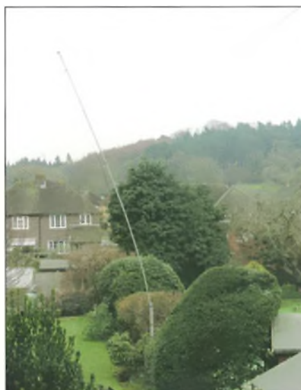
Fig. 5: 9.1m mast, leaning slightly due to offset antenna wires.
