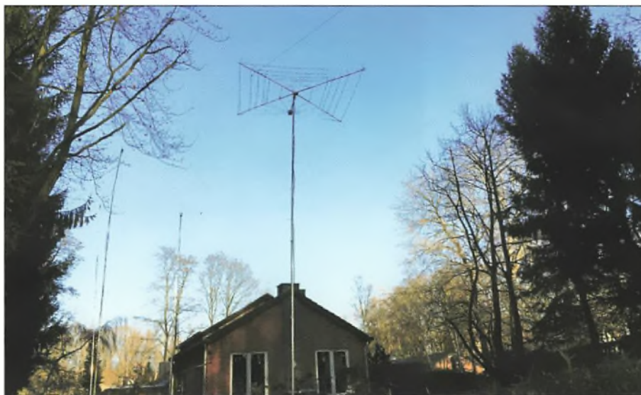
Fig. 3: The new CobWebb antenna at the QTH of Etienne OS8D.
