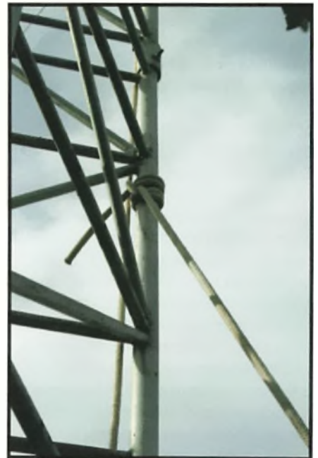
Fig. 14: The rope holding the author in the previous photo – a camel hitch around the leg of the second tower.
