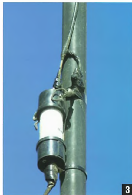
Fig. 2: (a) The classic, theoretical, figure-of-eight pattern of a standard dipole. (b) If the feeder radiates the pattern is more likely to be similar to this. Fig. 3: The W2AU balun connected at the lower end of the RG58 'CFR section'. The balun is secured to the Spiderbeam fibreglass pole with cable ties.
