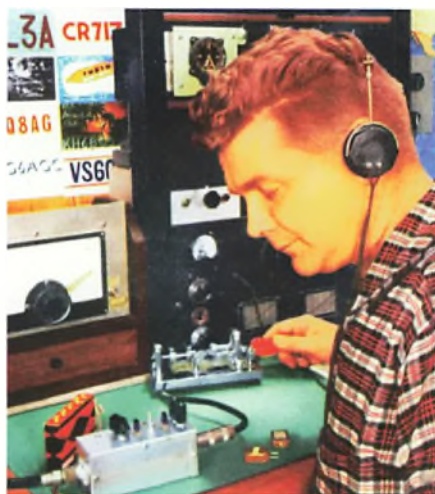
W10GU achieved the first transatlantic QSO with a 78mW transistor transmitter in September 1952.
