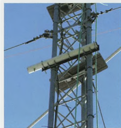
Fig. 4: Pulley Support Arm.
