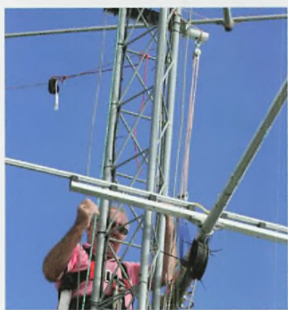
Fig. 5: Photo showing pulley arrangement.
