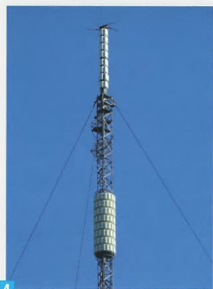
Fig. 1: Two VHF TV antennas of about 1960, still on a rooftop in 2019, along with a more modern UHF TV antenna. Fig. 2: (a) Shadow effect at VHF, 2(b) More extended shadow at VHF, 2(c), Shadow greater still at microwave frequencies. Fig. 3: The Stockland Hill UHF TV transmitter covers West Dorset, East Devon and the surrounding areas. Fig. 4: The main and reserve TV antennas on the Stockland Hill tower.
