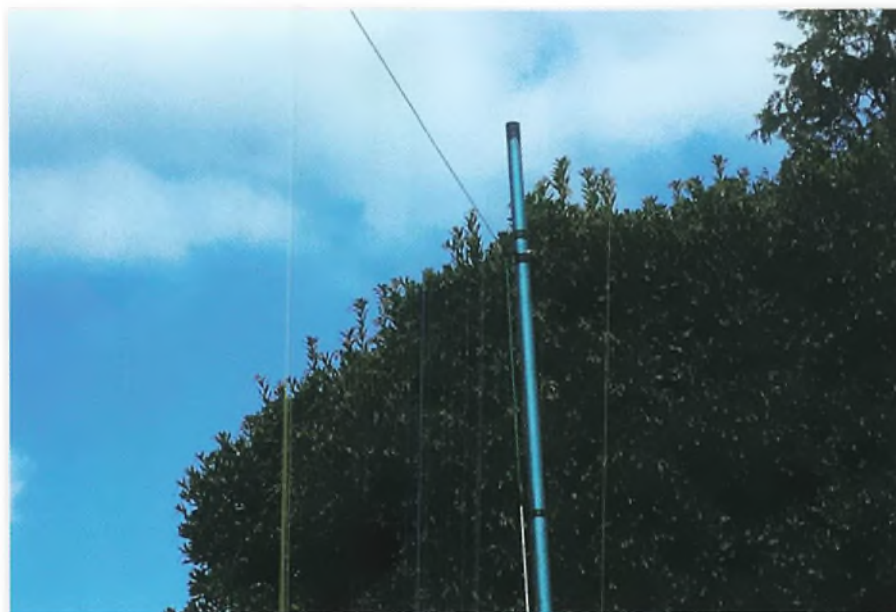
The wire reaching an end support pole. Note how the wire runs directly downwards for a short distance.
