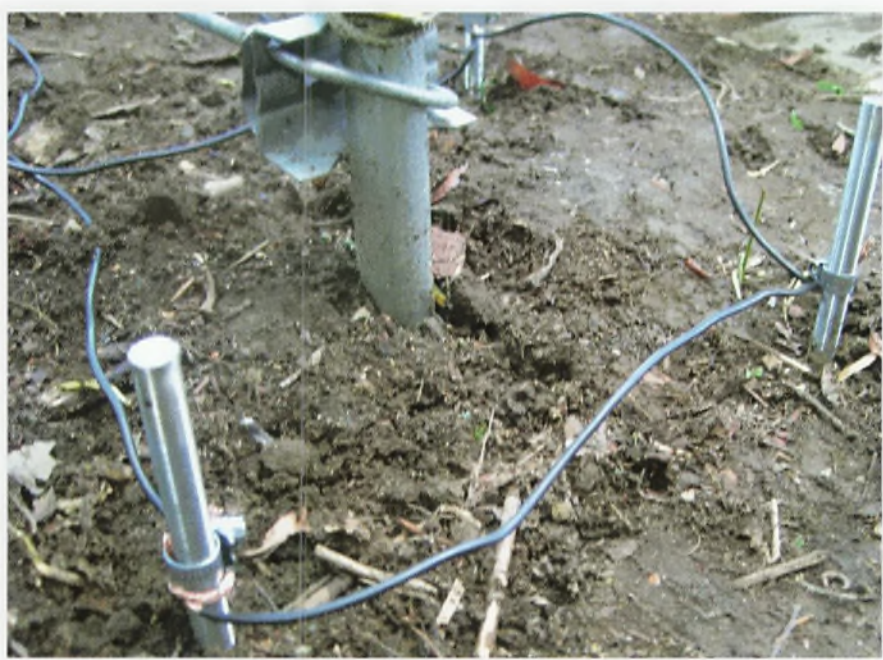
Fig. 6: 33ft of ground rods hammered in for G3JNB's new vertical.
