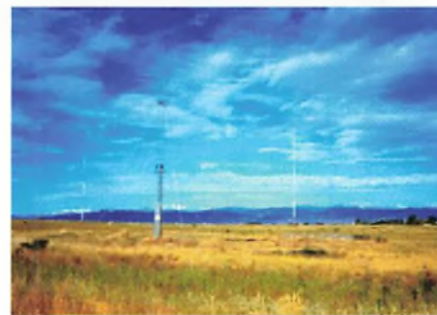
Fig. 2: The 15MHz antenna of WWV, a vertical dipole.
