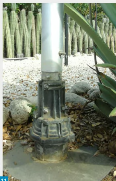
Fig. 9: The bolts on the bottom of the rotator that fix it to the rotator plate were very badly corroded (photo: Bert PJ4KY).
