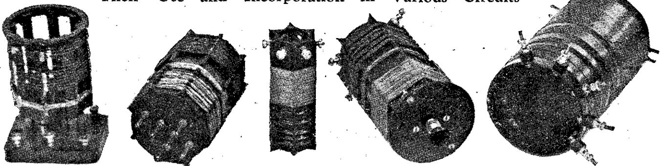
A set of home-made tuning coils. Reading from left to right the coils are: A short-wave tuner with 6-pin base; a broadcast tuner with 6-pin base; a smaller dual-wave tuner suitable for use in screen-grid receivers; a broadcast tuner with built-in wave-change switch, and another broadcast tuner for baseboard mounting. The first coil shown is wound on a skeleton former, the second, third, and fourth use ribbed ebonite formers, and the fifth is wound on a paxolin tube.
