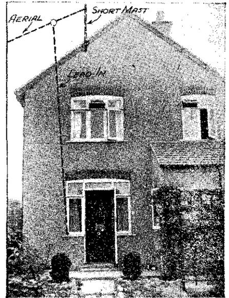
Fig. 2.—Using a short mast for anchoring the house end of aerial.
