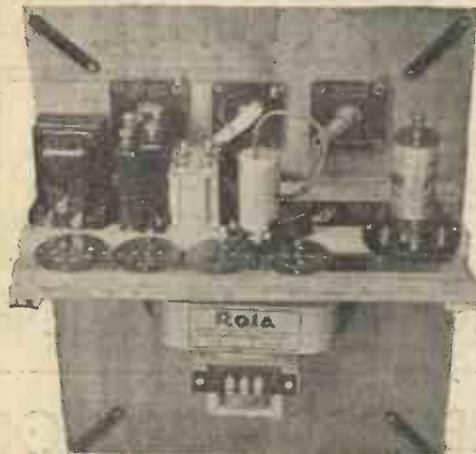
View showing the partly assembled receiver.
