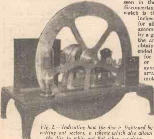
Fig. 2.—Indicating how the disc is lightened by cutting out sectors, a scheme which also allows the disc to whip out flat when revolving.
