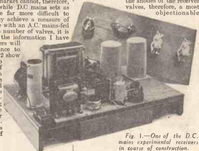
Fig. 1.—One of the D.C. mains experimental receivers in course of construction.
