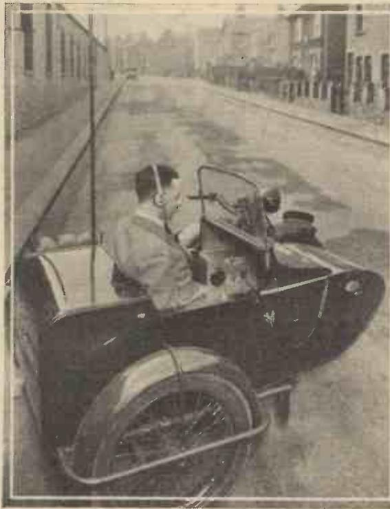
The above illustration shows a motor-cycle combination for police work fitted with a Marconi six-valve single-control police receiver operating with a short rod aerial.
