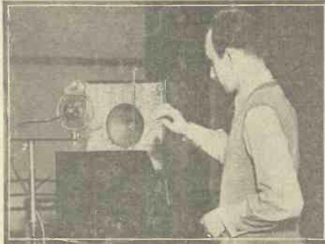
"His Master's Voice" have just issued the first records made by Martin Taubmann on the new *Electronde* instrument. He is seen recording four popular numbers at the H.M.V. studios. The musical notes from the *Electronde* are produced by moving the right hand to and fro from the upright rod. By pressing a switch held in the left hand the tone can be interrupted and the volume varied by pressing a pedal with one foot. The instrument has a nine octave range.
