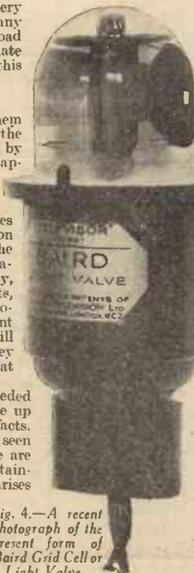
Fig. 4.—A recent photograph of the present form of Baird Grid Cellor Light Valve.
